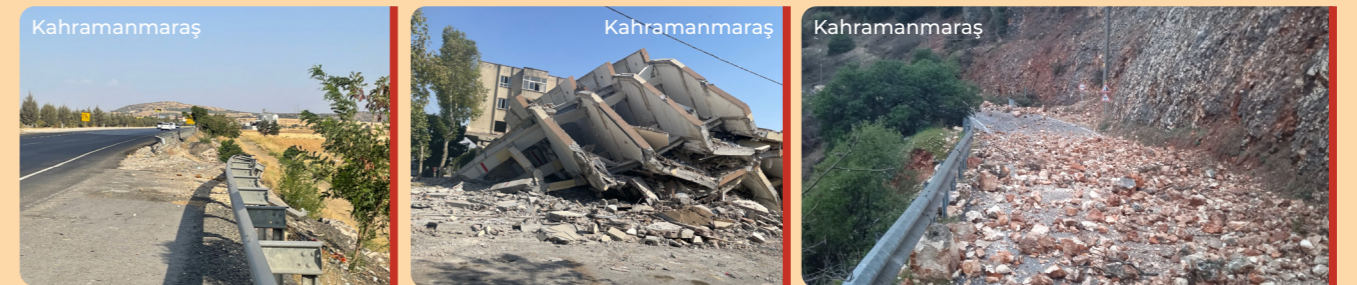
Road deformed by active fault
